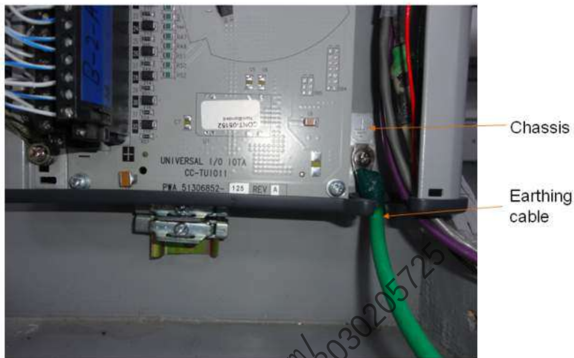
Figure 164: Grounding connections
